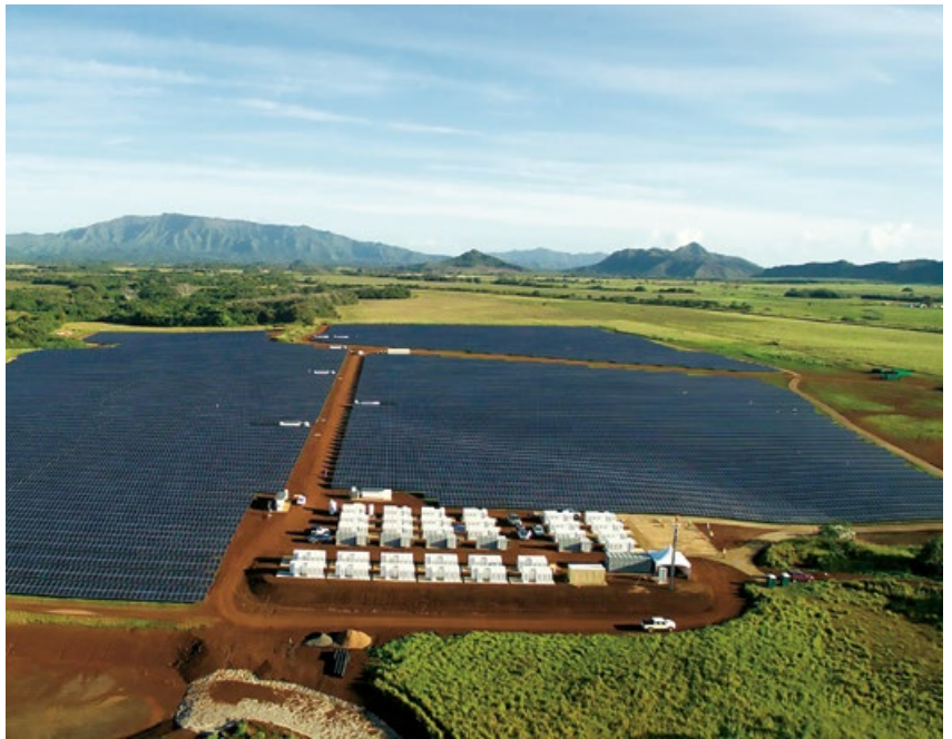
Pioneering project: On the Hawaiian island of Kauai, the first solar park with Tesla power packs is being built on a 26-hectare area that caches solar power.
