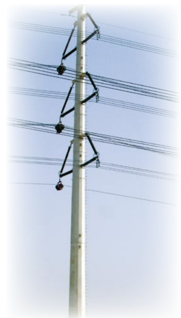
420 kV Insulated Crossarm
