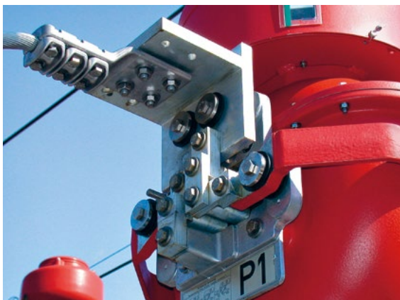
Figure 2: Protection against corrosion: Al Elast contact disks hermetically seal contact points
