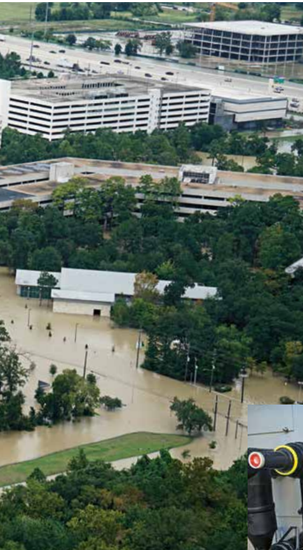
Flooded streets in Houston in the aftermath of Hurricane Harvey. Once the water subsided, the power grid was repaired – with the help of SICON screw connectors.
