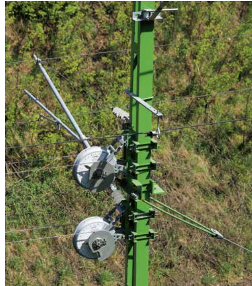
The compact TENSOREX C+ spring-tensioning system is the modern alternative to conventional wheel tensioning systems.
