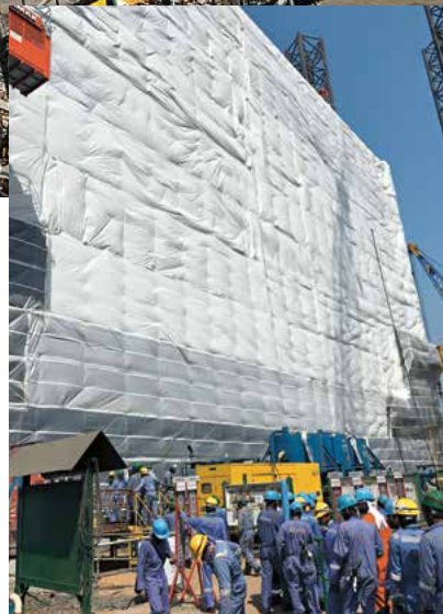
The platform in the port at Dubai: Working at over 40 °C.
