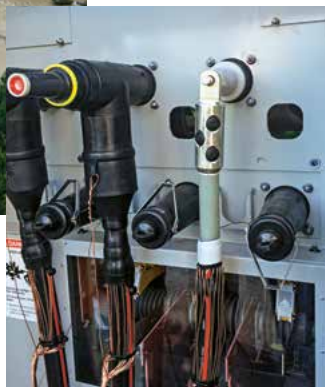
The right SICON connector for every application. Here as a contact element in the outer-cone plug.
