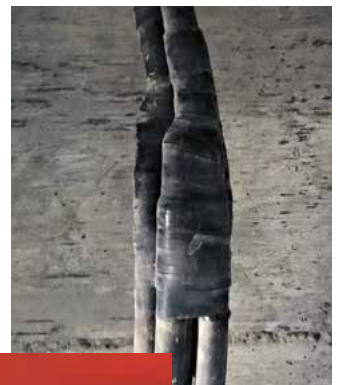
SICON branch connectors: The patented shear bolts break away burr-free and can be covered in heat shrink immediately after installation.
