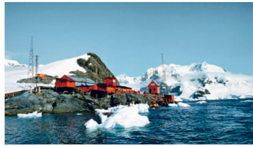
In remote places, transport costs for fossil fuels play an important role. Here, a CrossPower system pays off very quickly.
