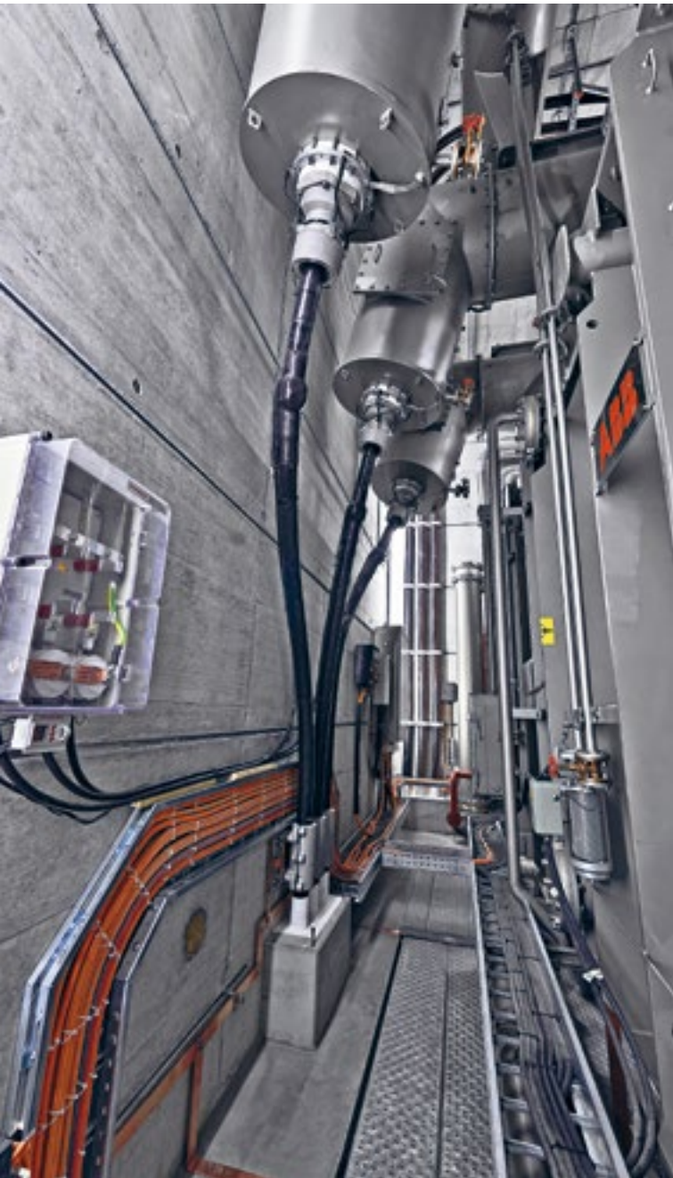
Touchproof under high voltage: Three cable connections to a 50-MVA transformer designed with encapsulated size 6 HV-CONNEX system for 170 kV as well as earthing isolator box for efficient screen treatment
