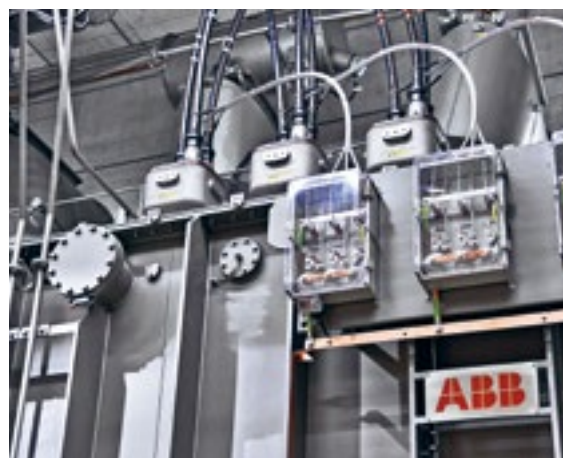
Extremely compact design from a single source: PFISTERER's new size 3 CONNEX transformer sockets (TAT) for up to 52 kV enable the multiple connection of vertically installed MV cables. The latest addition to the proven CONNEX system makes its debut at the Oerlikon substation – in conjunction with earthing isolator boxes and DSA-i3 continuous voltage indicators.
