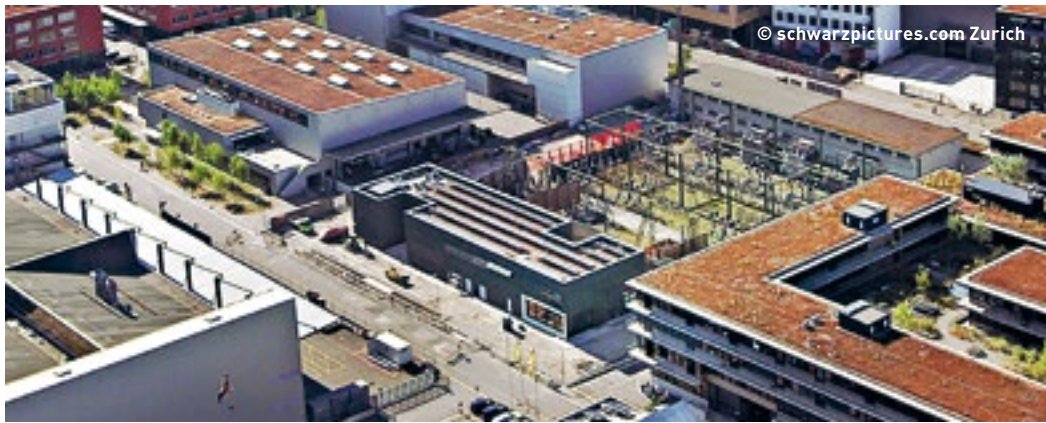
Smart savings: The new ewz Oerlikon substation was built in an urban area of Zurich and is located across three underground levels, directly below an ewz network base (center), which is also new. Together, the buildings take up visibly less space than the old air-insulated substation of the previous substation alone (behind new ewz network base).
