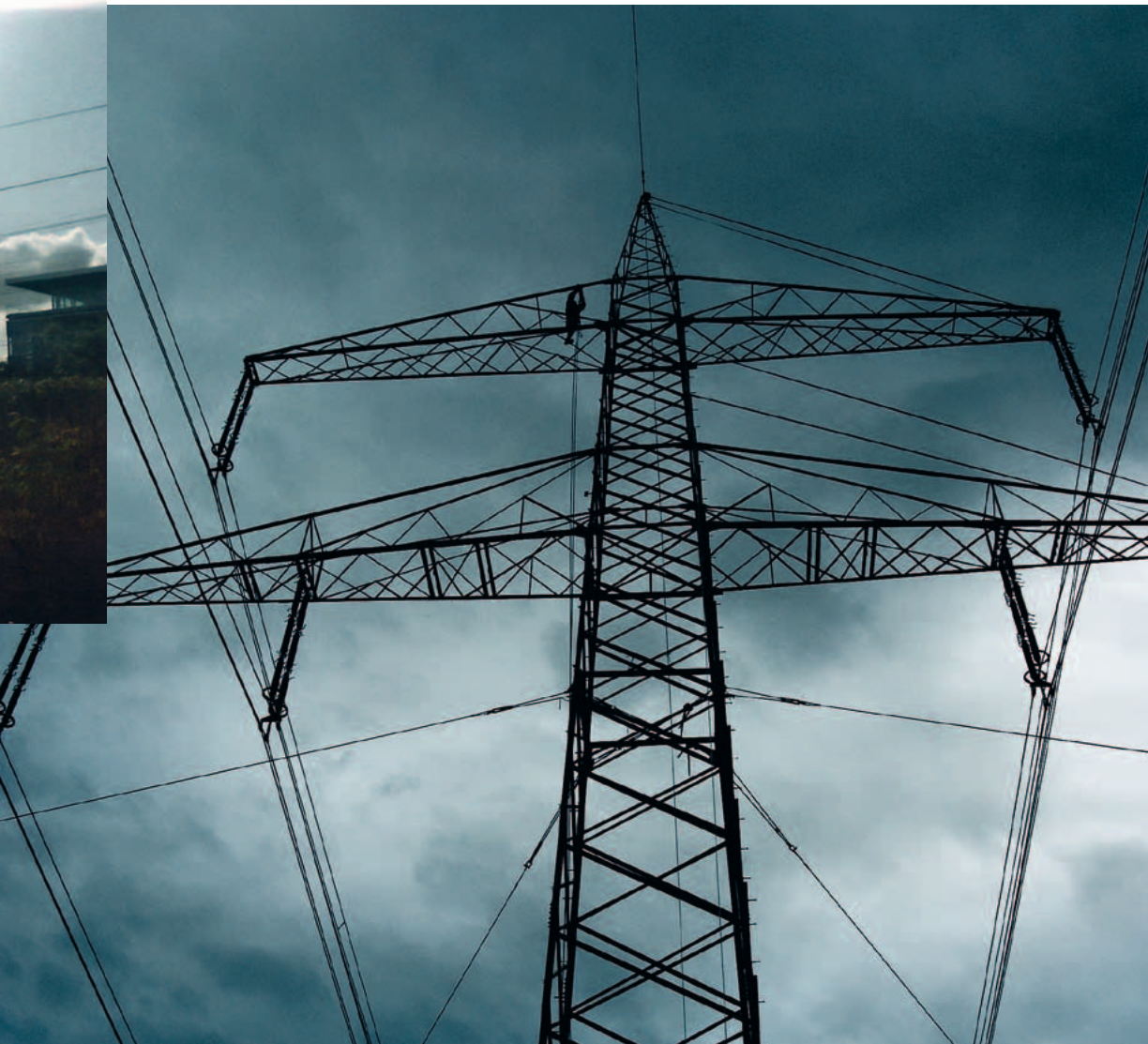
Figure 9: When performing voltage testing on overhead lines, atmospheric turbulence can “carry off” acoustic indicator signals. Very bright sunlight can blind users equally whether they are in an elevated position or on the ground. These and other unfavorable environmental influences are not uncommon during voltage testing, which explains the crucial importance of signal design with regard to voltage detectors.
