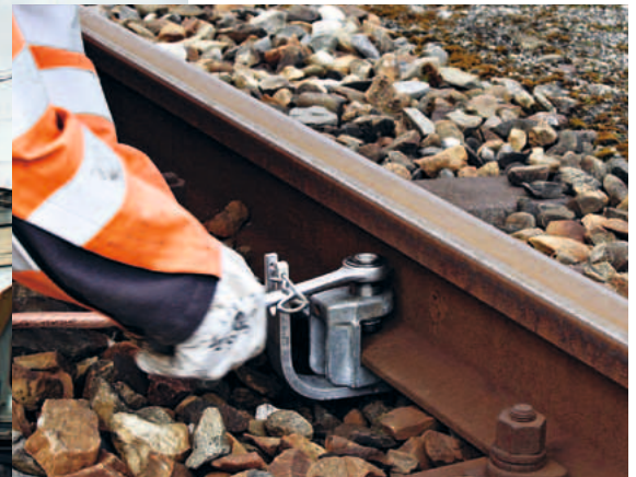
Load-bearing rail earthing clamps ensure that the earthing and short-circuit set is held securely on the track.
