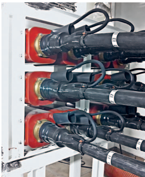
Field-tested predecessor: CONNEX connection joints of size 3 in use at high sea, such as here on an offshore substation.
