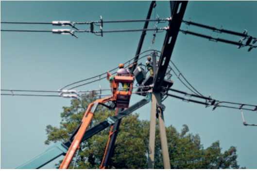
Installation of PFISTERER products at the changeover from the new Verbois substation to the existing 245 kV substation (left image) and after installation (right image): Post insulators standing on the portal; the high-load terminal chain is projecting horizontally toward the left.
