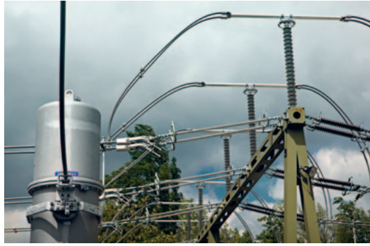
Installation of PFISTERER products at the changeover from the new Verbois substation to the existing 245 kV substation (left image) and after installation (right image): Post insulators standing on the portal; the high-load terminal chain is projecting horizontally toward the left.
