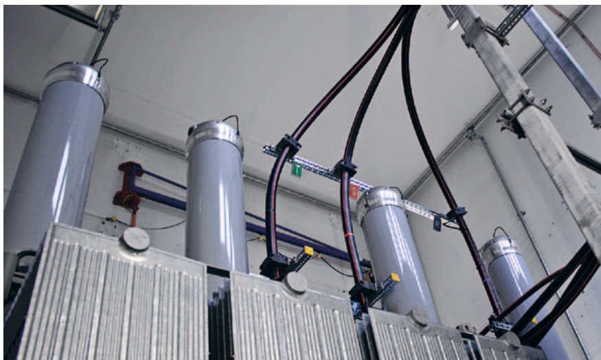
Visible advantages of the pluggable, solid-material insulated CONNEX system as compared to air insulated solutions: You do not need to adhere to minimum clearances or install busbar platforms on the transformers and substations.
