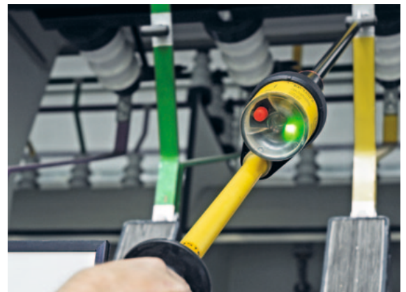
Voltage tester KP-detector 5 gives a green light for maintenance work.
