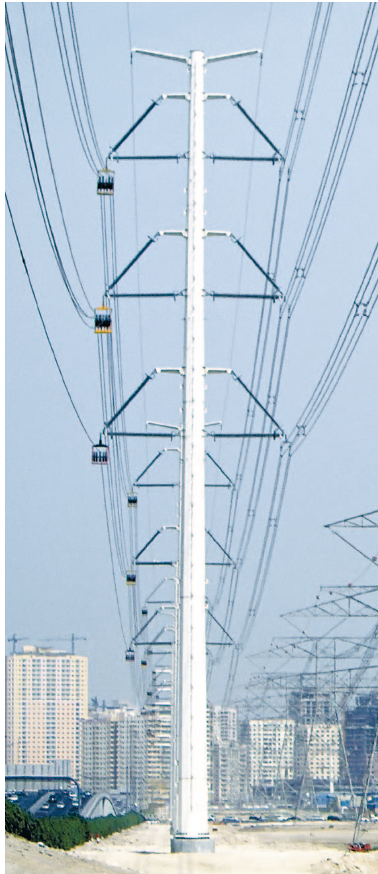
Experience for development work: PFISTERER insulator crossarm for 420-kV compact cables in Dubai (in upper left image) and in the Netherlands (see computer graphic at the right). The insulator crossarm unifies the insulation function and the load-bearing pole arm function. This double function creates their special construction of at least two insulators, one angled tension insulator and one horizontal or slightly tilted pressure insulator.
