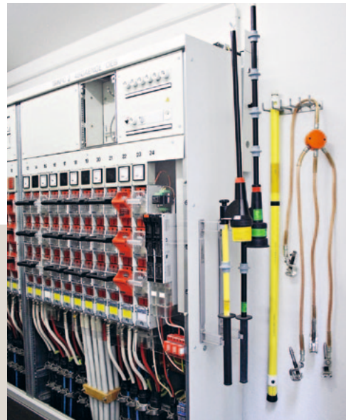
Voltage testers and earthing accessories from PFISTERER within reach for distribution with PFISTERER connecting blocks
