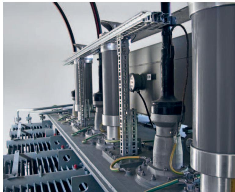
HV CONNEX surge arresters installed in a power transformer.
