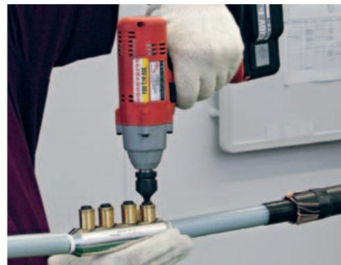
Only certain impact wrenches are suitable for the installation of shear off bolts.
