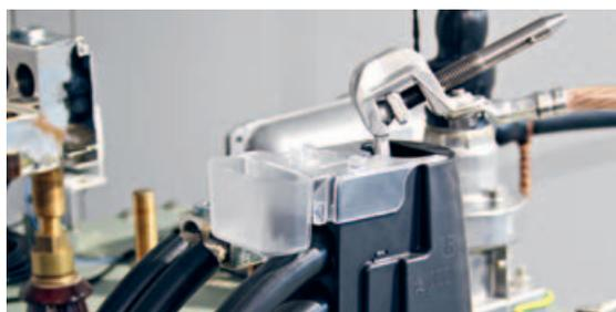
This can be easily opened with an insulating pole from a safe distance so that you can easily reach the protruding fixed ball point for connecting the earthing device from all sides.
